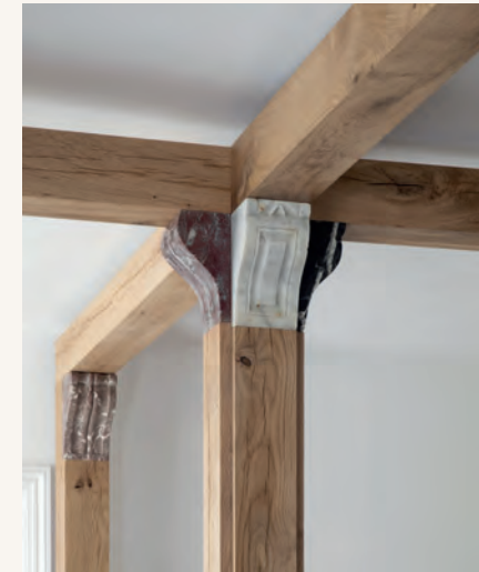
© Amor Immeuble - DNL gallery © Amor Immeuble
